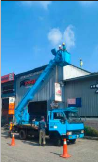
Roof Condition Assessment
