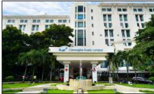
Gleneagles Hospital Level 5 Refurbishment (MEP Engineering Design & Installation Works) • Kuala Lumpur
