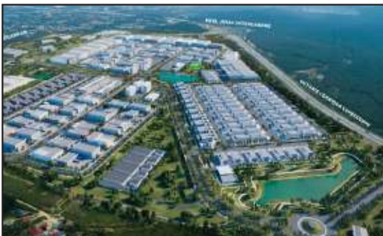
Sime Darby Elmina Business Park 60 Units of Twin Factories (TNB SSU, External Infrastructure, Electrical Works) • Rawang
