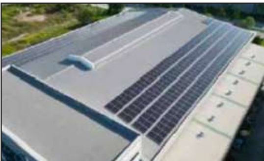
Location: Klang, Selangor System Size: 190.92kWp
