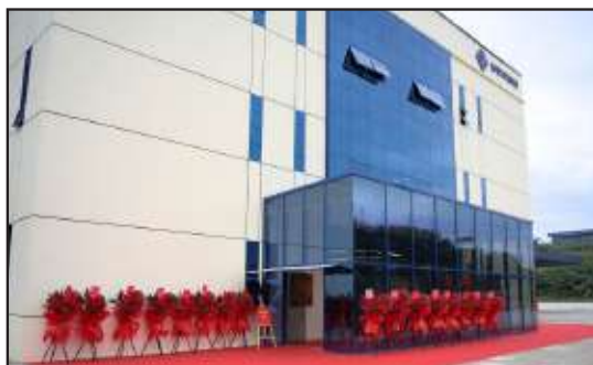
Weyoung Switchgear Manufacturing Factory Electrical Works • Kulai
