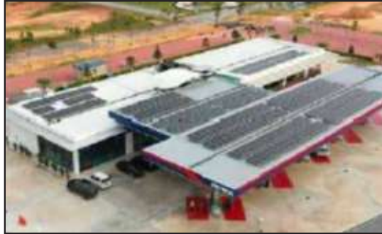
Location: Sendayan, Negeri Sembilan System Size: 112.84kWp
