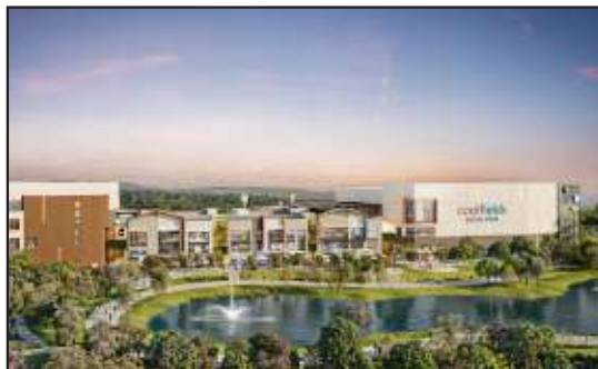
KLK Bandar Seri Coalfields Retail Park Block E1 & E2 (External Compound Lighting & Building Electrical Works) • Sg Buloh
