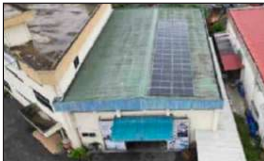
Location: Klang, Selangor System Size: 18.87kWp
