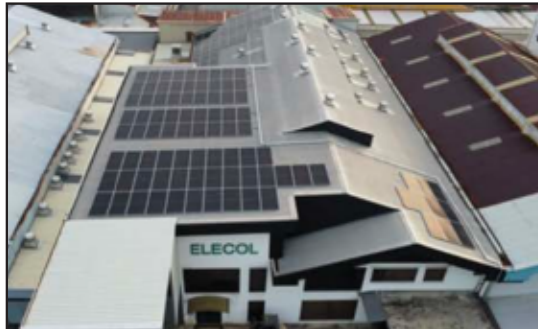
Location: Serdang, Selangor System Size: 84.16kWp
