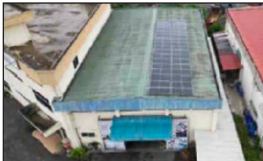
Location: Klang, Selangor System Size: 18.87kWp
