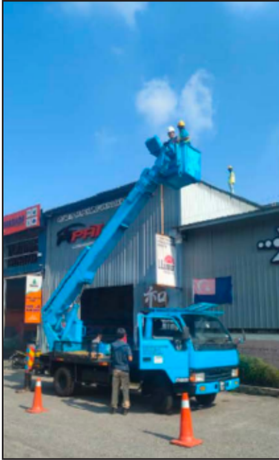
Roof Condition Assessment
