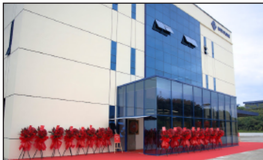
Weyoung Switchgear Manufacturing Factory Electrical Works • Kulai
